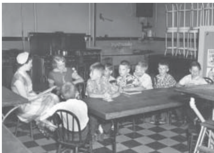
Original basement kitchen being used for Sunday School class.
