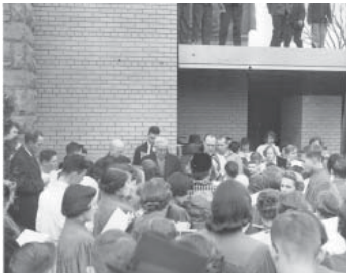
Laying of cornerstone of Parish Education unit - 1955.
